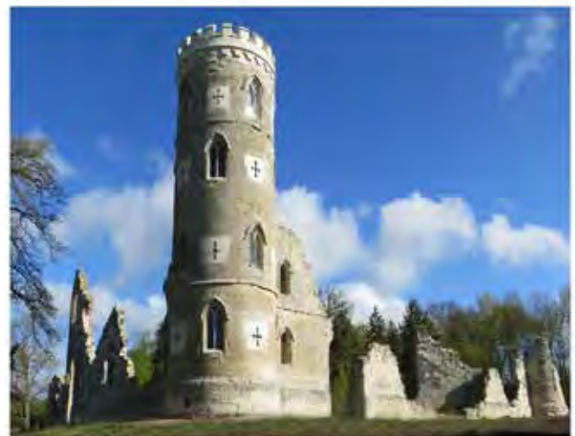
Wimpole Gothic Tower after conservation of all masonry and replacement of crenellations and arrow slits
