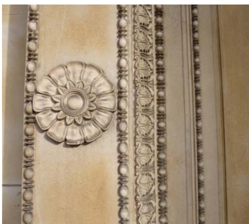
① Detailed coade-type mouldings at St Pancras New Church, London, a building designed by William Inwood and son Henry William Inwood, completed in 1822
