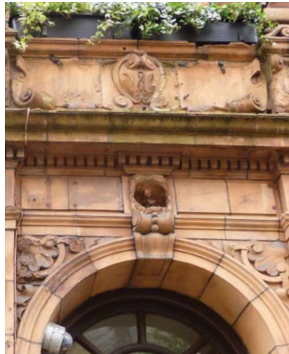
5 Terracotta with drill holes that may or not be filled afterwards, and if they are it is often done poorly
