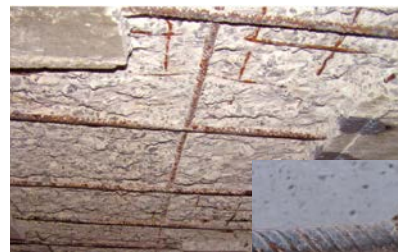
❷ All the steel should be covered to the right depth, not just the main bars
