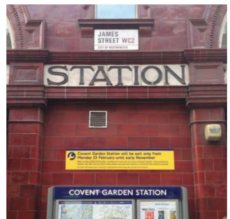
③ The grade II listed Covent Garden underground station, 1907, designed by architect Leslie Green. Its tiles use twice-fired oxblood faience, manufactured by the Leeds Fireclay Company
