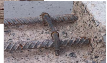
❷ All the steel should be covered to the right depth, not just the main bars
