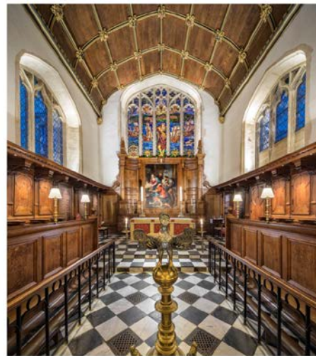
Corpus Christi College Chapel Oxford, after major restoration including plaster work, decorative timber repairs, polychrome & gilding ceiling ribs, floor repairs & stone monument repairs.
