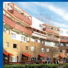
Roof refurbishment and canopies Byker Wall Estate, Newcastle-upon-Tyne
