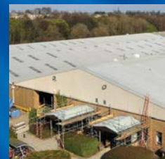
Lightweight GRP over-roofing Water company depot, Yorkshire
