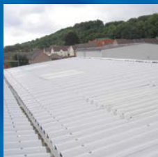
Simpler, more cost-effective roof refurbishment Industrial Unit, Wiltshire
